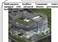
Outer shell structural system with no use of welding and employing coupled vibration control technique (or suspension structure)
