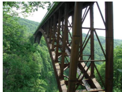
Weathering steel bridge
