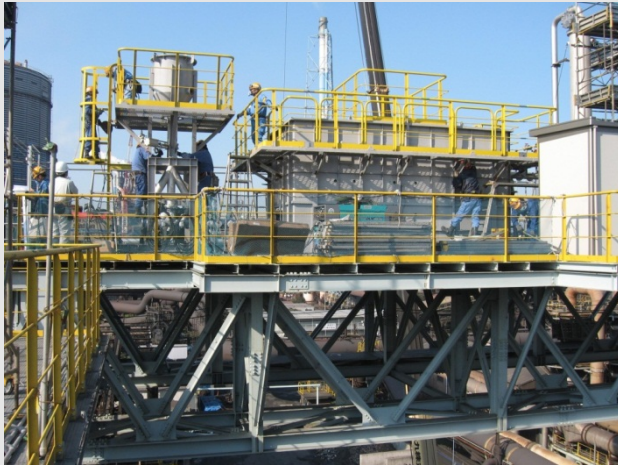
Catalytic large reactor (shown during installation)
