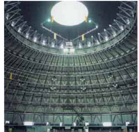
Photo 1 Inside view of Sun Dome Fukui
