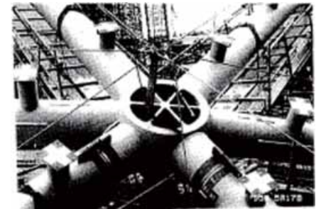
Installation of node section
