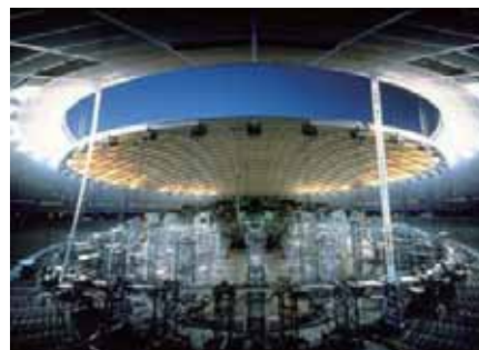
Lift up of the roof in the second stage of construction
