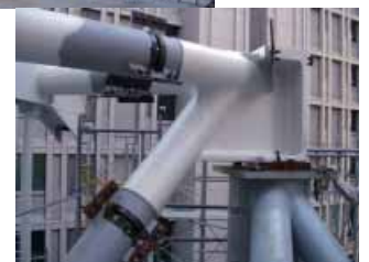
Edge of ship-shaped truss
