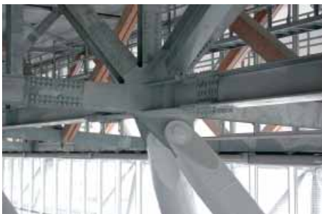
Cast steel member adopted for the truss beam cross section
