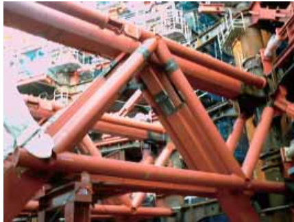
Fig. 4 Damper for bending deformation
