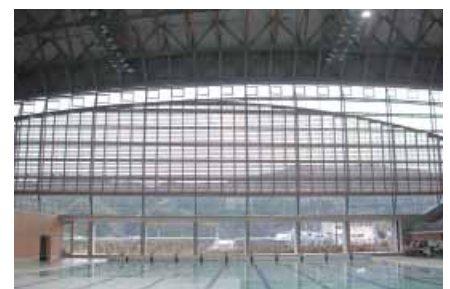
Vierendeel steel truss used for wall
