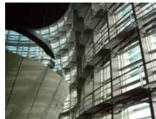
Glass façade with a three-dimensional curved surface
