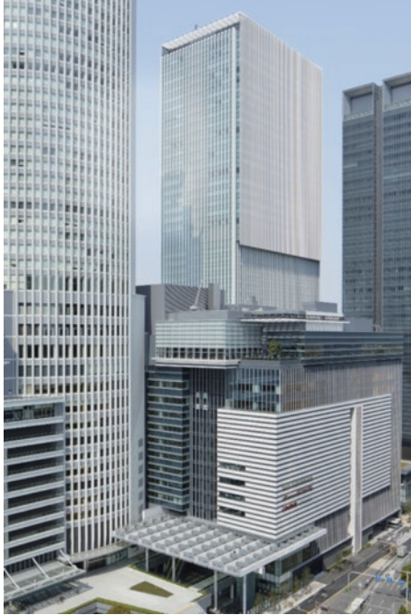
Photo 1 Appearance of JR GATE TOWER
