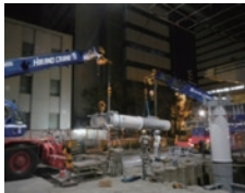
Photo 2 Erection of lower column
