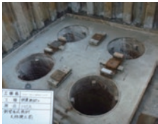
Photo 1 Installation of erection platform on leveling concrete
