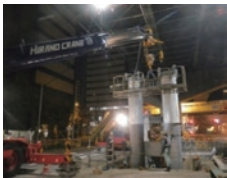
Photo 3 Erection under low overhead clearance
