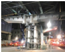
Photo 4 Erection using two 60-ton cranes
