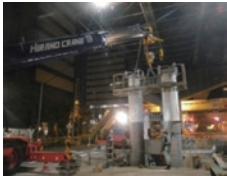
Photo 3 Erection under low overhead clearance
