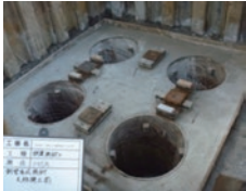
Photo 1 Installation of erection platform on leveling concrete
