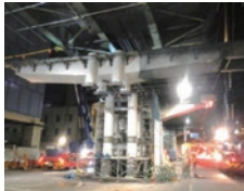
Photo 4 Erection using two 60-ton cranes
