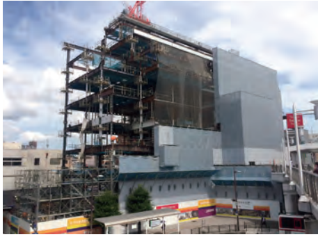
Photo 4 Steel structure construction
