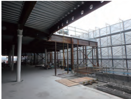
Photo 6 Building structure employing heavy-wall seamless steel tube
