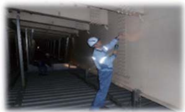
Photo 3 Interior of multi-function corrosion-protection deck
