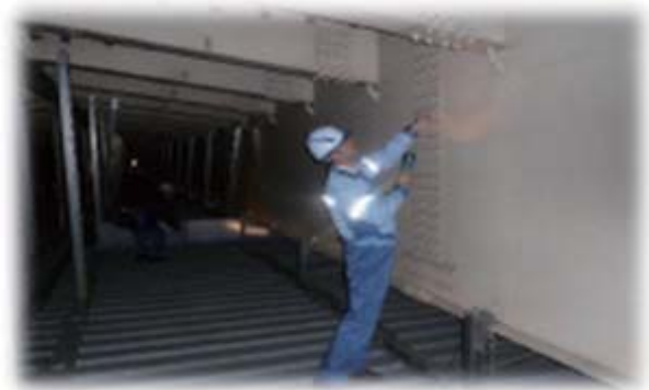
Photo 3 Interior of multi-function corrosion-protection deck
