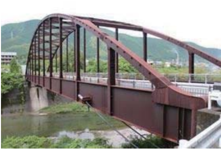
Photo 2 Special-type bridges constructed using weathering steel
