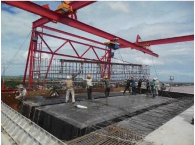
Photo 7 Prefab rebars for cross beam
