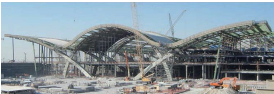
Photo 2 Installation of arch column steel framing
