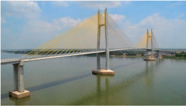
Photo 1 Full view of Tsubasa Bridge
