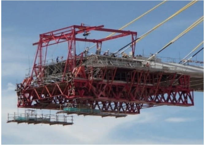
Photo 6 Form traveler for 8 m blocks
