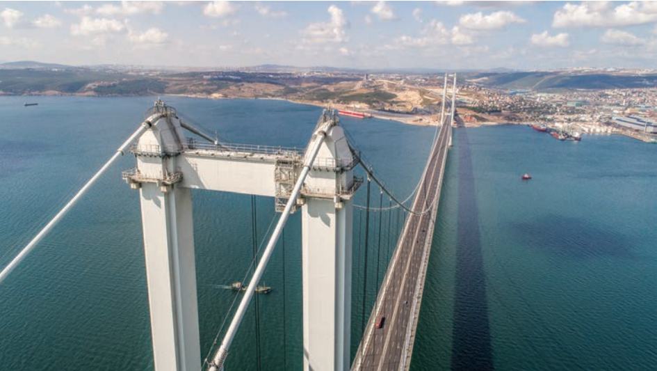
Photo 6 View at tower top
