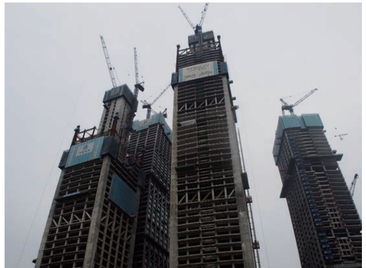
Raffles City Chongqing project underway
