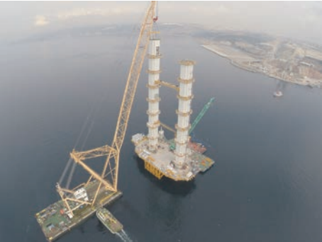
Photo 3 Tower block erection by floating crane
