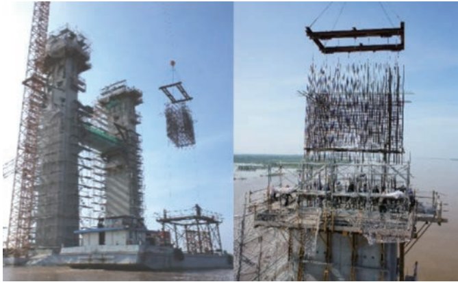
Photo 5 Prefab rebar for tower
