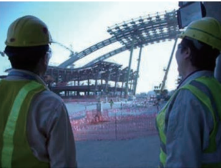
Photo 3 On-site confirmation of arch column steel framing by engineers
