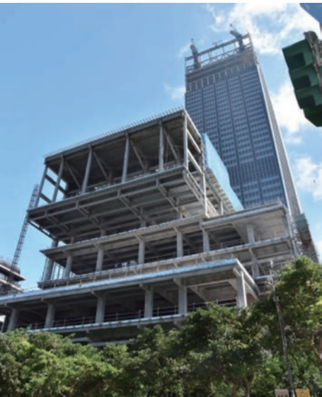
Photo 3 Erection of retail building
