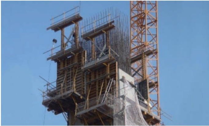
Photo 4 Jumping form system
