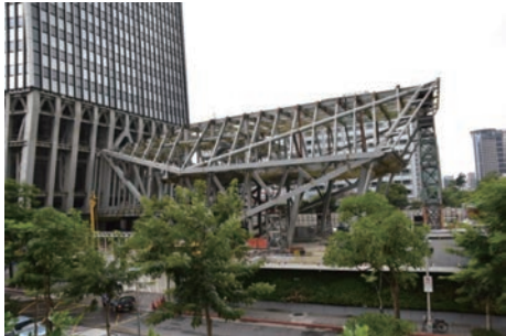
Photo 5 Erection of cultural building
