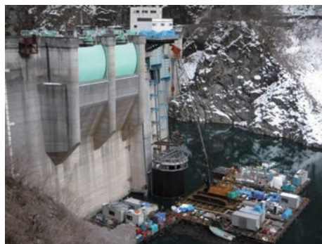
Photo 2 Installation of gate leaf (movable frame)
