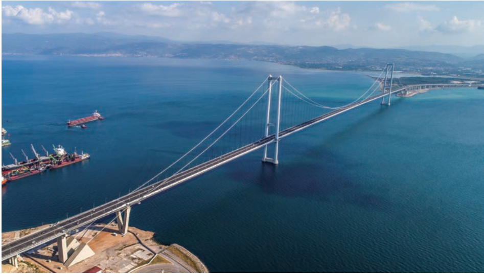
Photo 1 Aerial view of Osman Gazi Bridge
