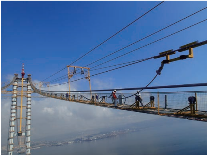
Photo 4 Main cable erection by PPWS method
