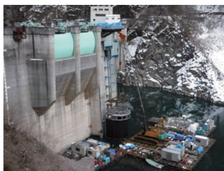
Photo 2 Installation of gate leaf (movable frame)
