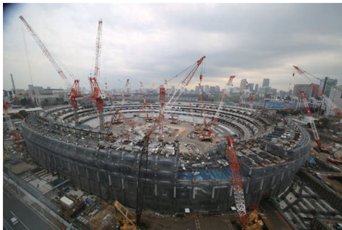
Construction is proceeding of the New National Stadium for the Tokyo 2020 Olympic and Paralympic Games (as of February 2018).
