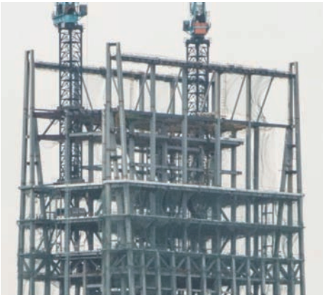
Photo 2 Erection of topmost section of office tower*
