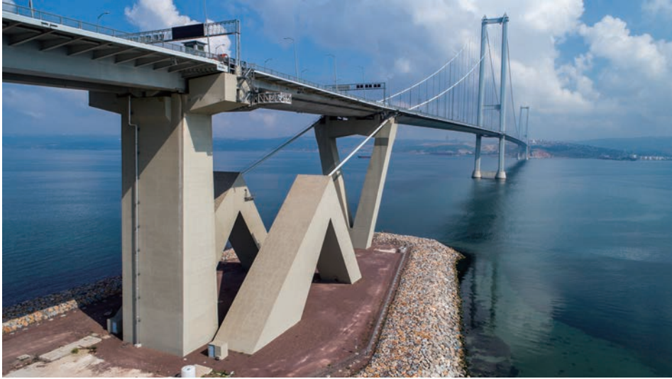
Photo 2 South anchorage area and the bridge
