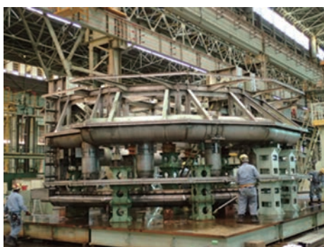
Photo 1 Factory temporary assembly of gate leaf (movable frame) employing SUS821L1
