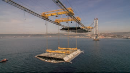
Photo 5 Deck erection by lifting device
