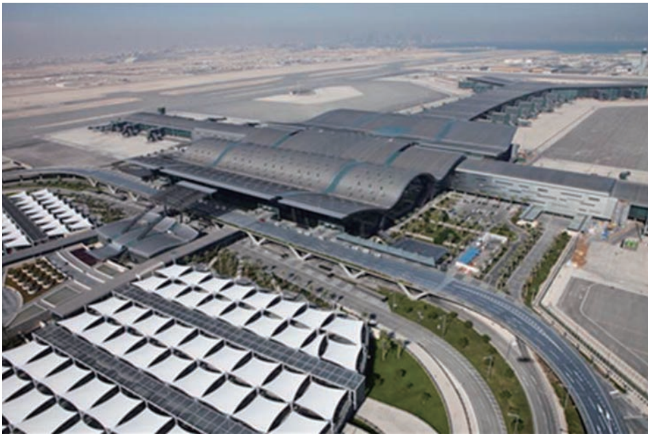
Photo 1 Full view of Passenger Terminal of New Doha International Airport in Qatar
