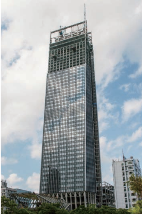
Photo 1 Erection of office tower*
