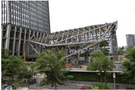
Photo 5 Erection of cultural building
