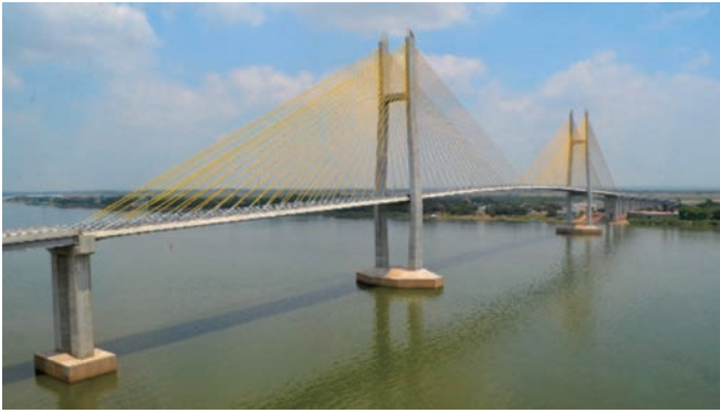
Photo 1 Full view of Tsubasa Bridge
