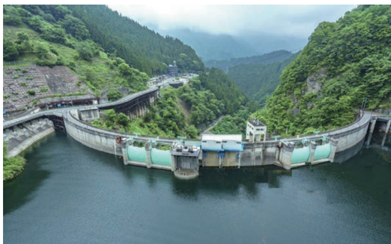
Photo 3 Full view of Futase Dam after completion of selective water intake facility
