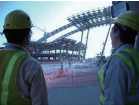
Photo 3 On-site confirmation of arch column steel framing by engineers
