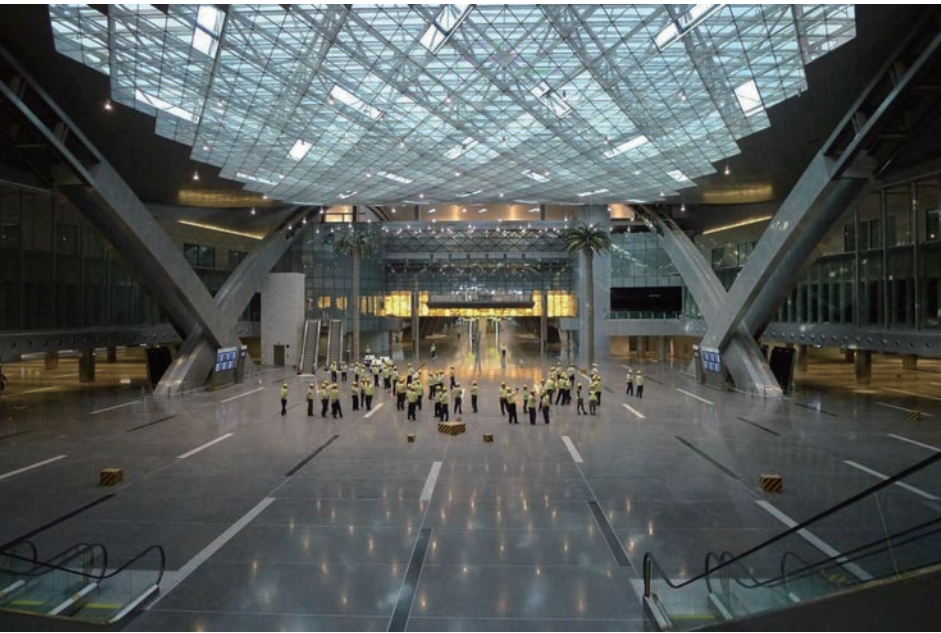
Photo 4 Top light of main terminal building
