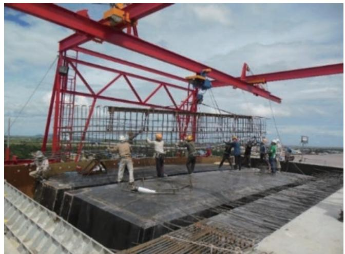
Photo 7 Prefab rebars for cross beam
