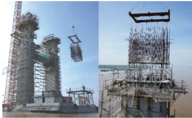
Photo 5 Prefab rebar for tower
