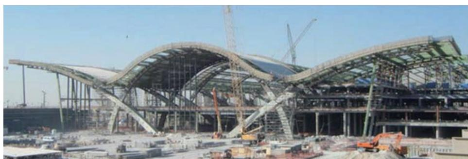
Photo 2 Installation of arch column steel framing
