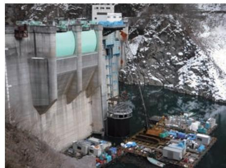
Photo 2 Installation of gate leaf (movable frame)
