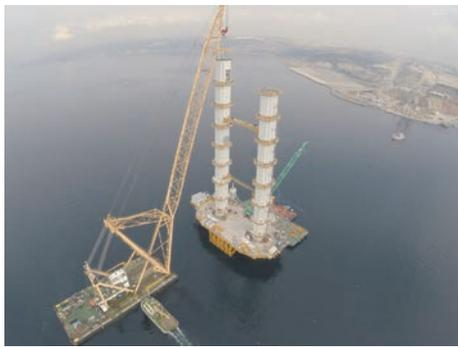
Photo 3 Tower block erection by floating crane
