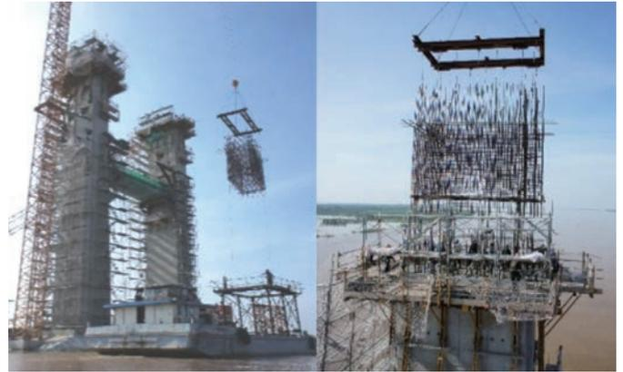
Photo 5 Prefab rebar for tower
