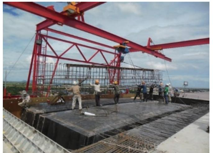
Photo 7 Prefab rebars for cross beam
