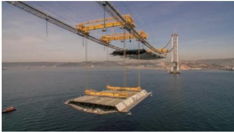
Photo 5 Deck erection by lifting device
