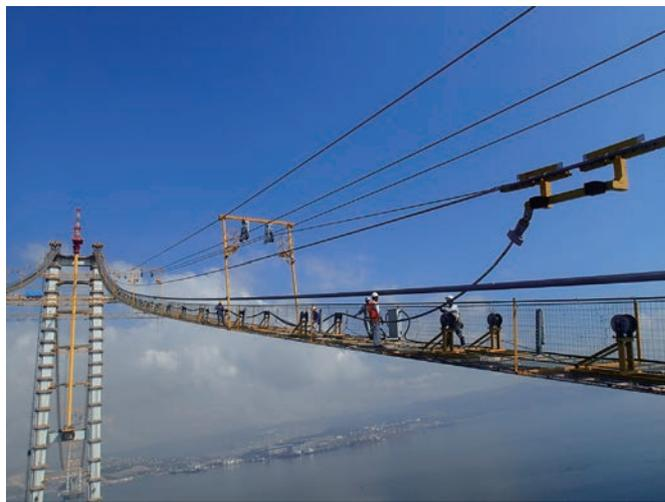
Photo 4 Main cable erection by PPWS method
