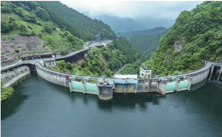
Photo 3 Full view of Futase Dam after completion of selective water intake facility
