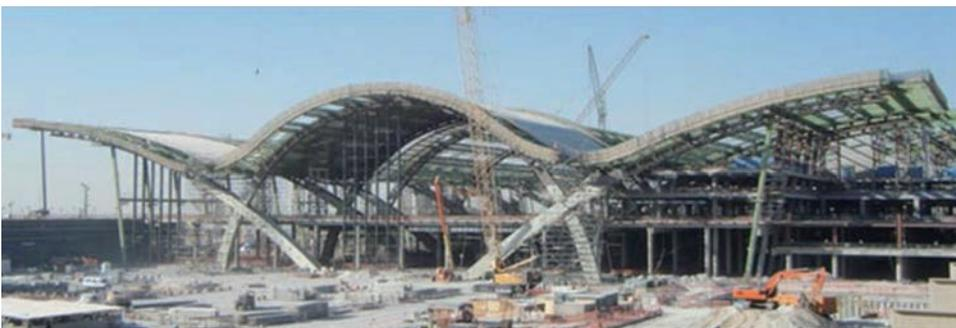
Photo 2 Installation of arch column steel framing
