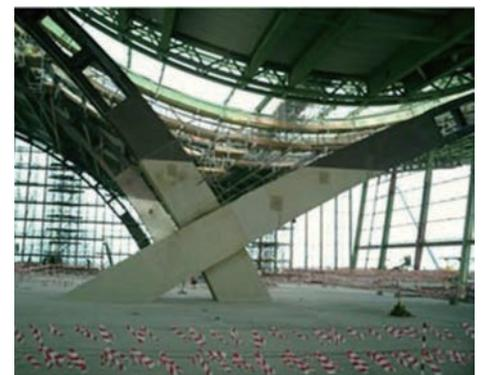
**Fig. 1 Installation Plan for Arch Column Steel Framing**
