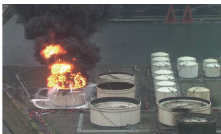
Photo 2 Fire of crude and naphtha tanks by long-period seismic motion (2003 Tokachi-oki earthquake)
