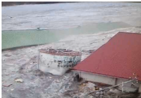
Photo 4 Floating out of oil tanks into the sea by the tsunami (2011 East Japan earthquake)
