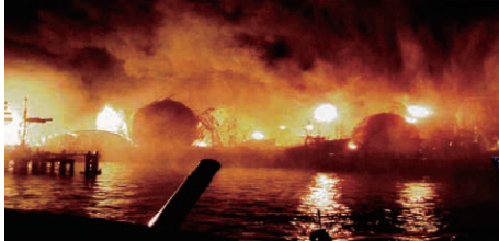
Photo 1 Explosion and fire of 17 spherical LPG tanks (2011 East Japan earthquake)
