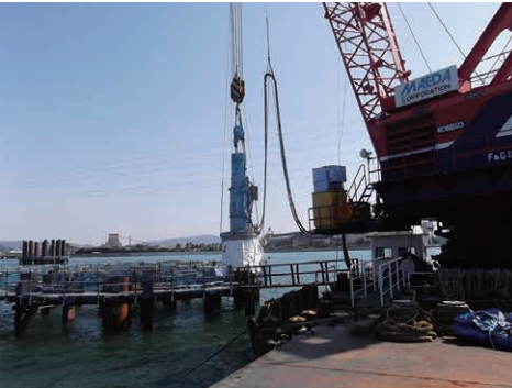
Photo 1 Condition of dynamic loading testing
