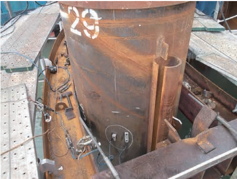
Photo 2 Condition in which sensors are pasted on test pile
