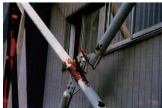
Fracture of brace joint
