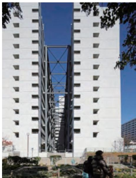
Photo 1 Kawaramachi housing after seismic retrofitting
