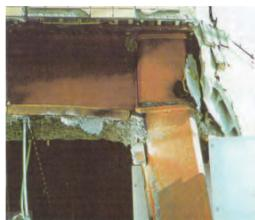
Fracture of column-beam connection
