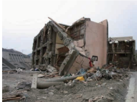
Photo 3 Building that overturned due to tsunamis
