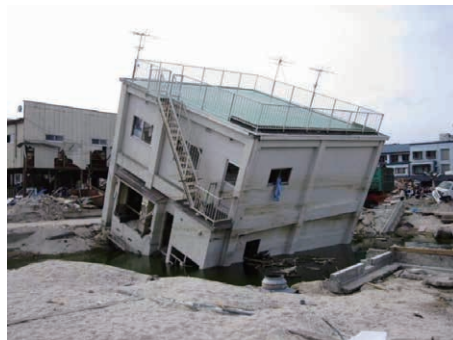
Photo 4 Building that inclined due to scouring
