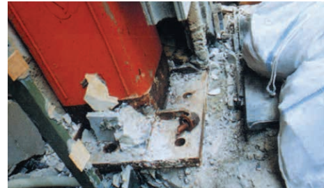
Fracture of anchor bolts of column base to cause dislocation of column
