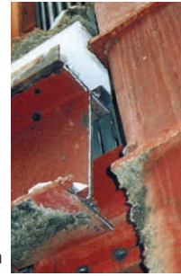
Fracture at beam end that occurred prior to its sufficient deformation
