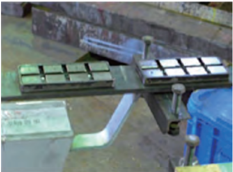
Photo 7 Magnet at anode-affixed section in cathodic protection method
