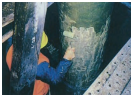
Photo 3 Underwater cured-type coating (coating of putty-state coat)
