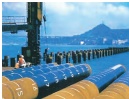
Photo 2 Polyethylene coating (black section: polyethylene)
