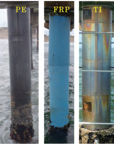
Photo 5 Appearance of protective cover of pet-rolatum coating method
