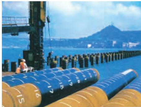
Photo 2 Polyethylene coating (black section: polyethylene)
