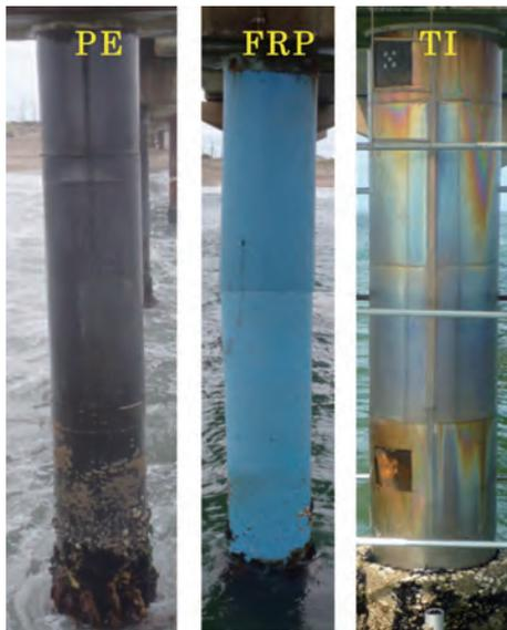
Photo 5 Appearance of protective cover of petrolatum coating method
