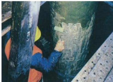
Photo 3 Underwater cured-type coating (coating of putty-state coat)
