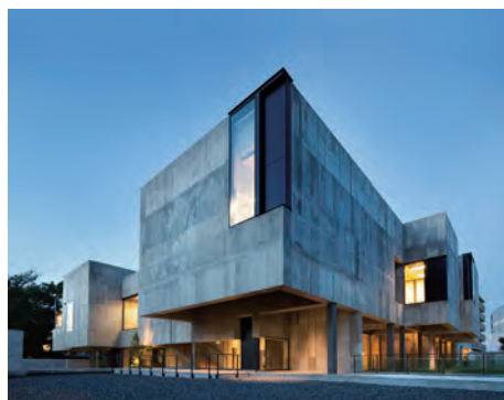
Photo 4 No. 1 Building of Toho Gakuen Chofu Campus
