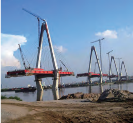
Photo 2 View of construction by cantilever erection
