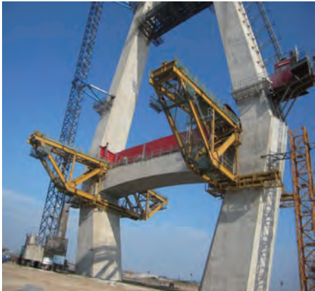
Photo 1 View of construction by inclined bent
