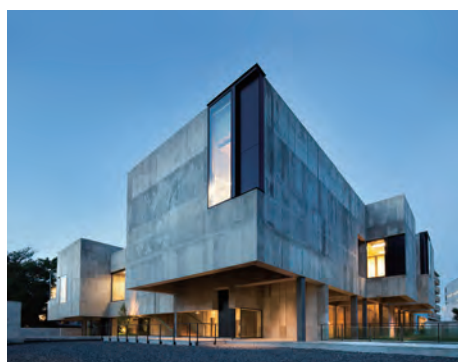
Photo 4 No. 1 Building of Toho Gakuen Chofu Campus
