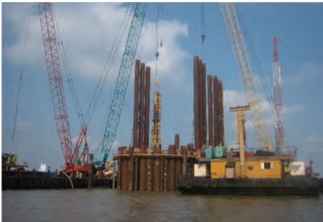
Photo 3 SPSP installation
