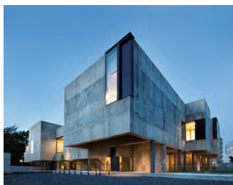
Photo 4 No. 1 Building of Toho Gakuen Chofu Campus
