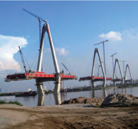
Photo 2 View of construction by cantilever erection
