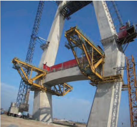
Photo 1 View of construction by inclined bent
