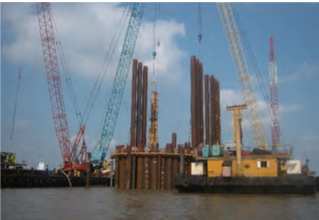
Photo 3 SPSP installation
