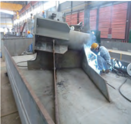
Photo 4 Steel fabrication works
