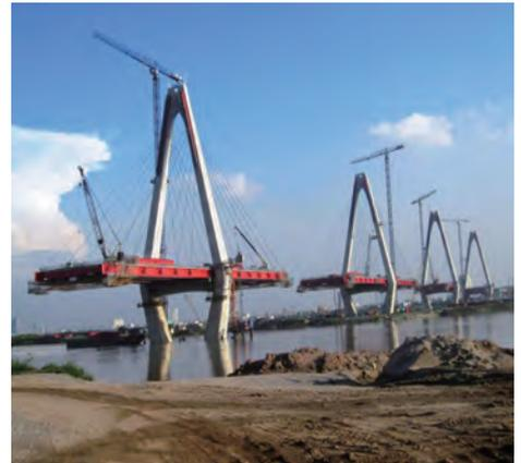
Photo 2 View of construction by cantilever erection
