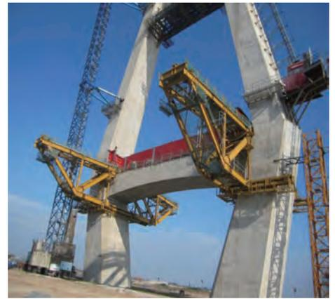
Photo 1 View of construction by inclined bent
