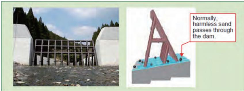
**Fig. 11 Impermeable Steel Dam to Block Sand**
