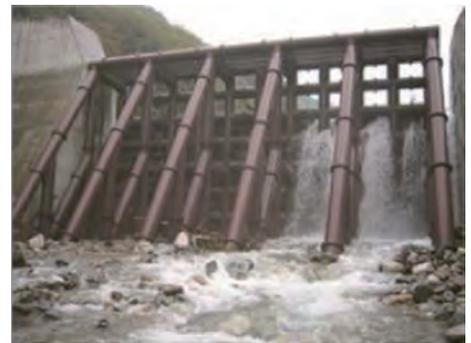
Shift-type structures is designed considering the ecosystem, which does not disrupt river flow.
