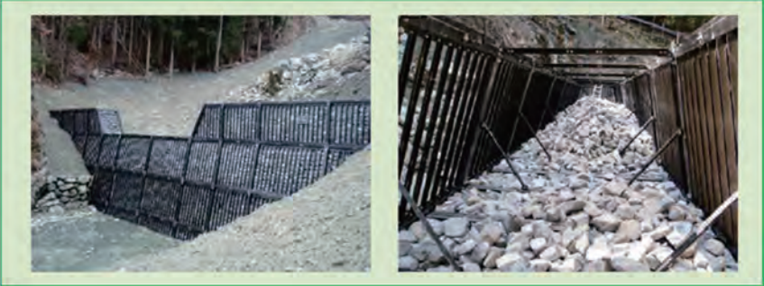
Fig. 11 Impermeable Steel Dam to Block Sand
