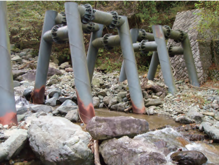
Photo 2 Slit dam as a case of infrastructural stock
