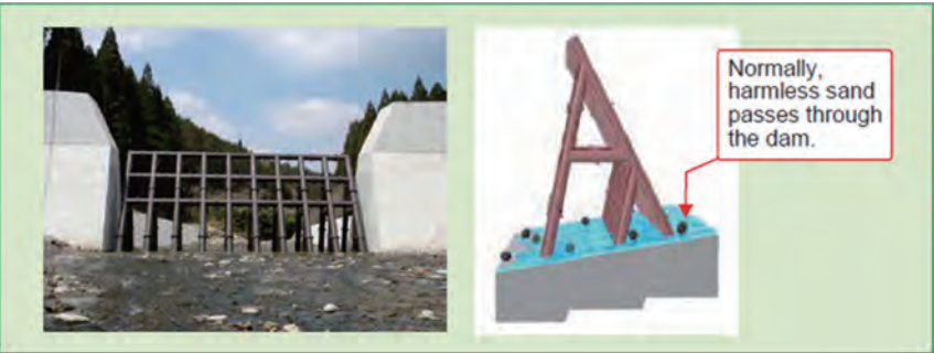
Fig. 10 Water-permeable Steel Dam to Prevent Sand Buildup
