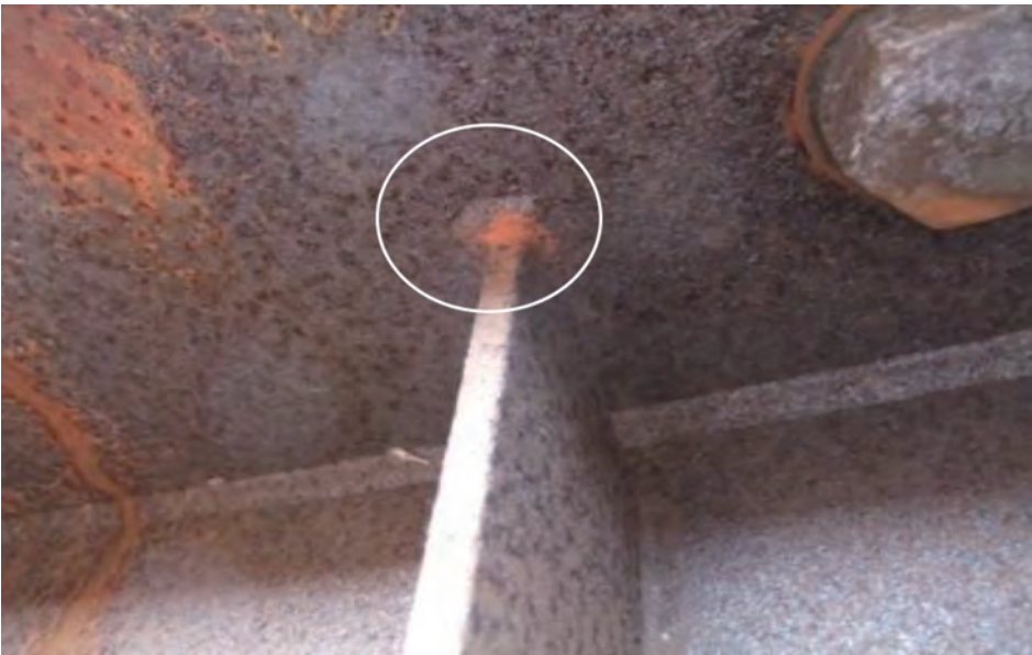
Photo 3 Fatigue crack
