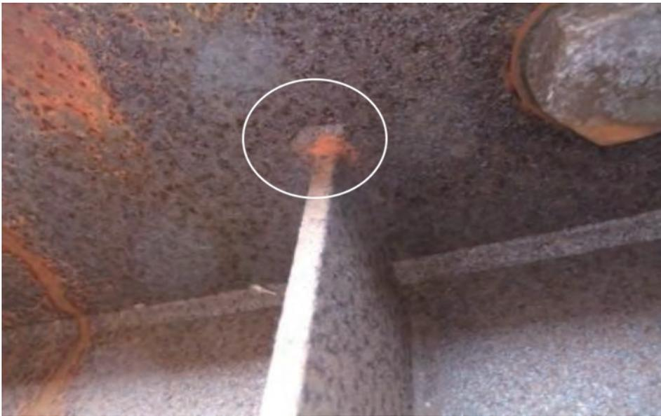
Photo 3 Fatigue crack
