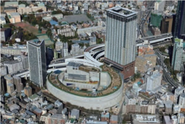
Photo 1 Full view of Ohashi Junction
