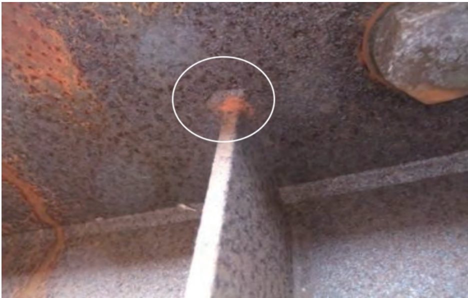
Photo 3 Fatigue crack
