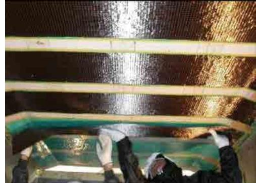
Photo 8 Reinforcement of RC slab with carbon-fiber sheet (sheet is pasted in the direction rectangular to slab; coating is provided to prevent deterioration of epoxy resin)
