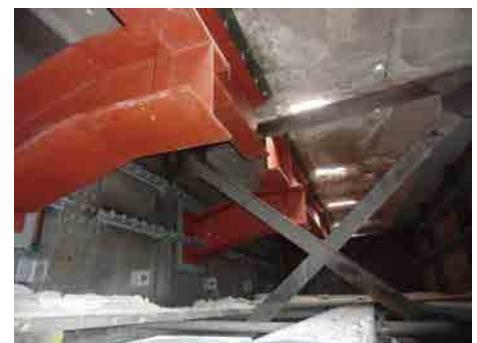
Photo 3 Bracket for use for RC slab reinforcement
