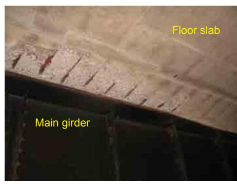
**Photo 2 Exposure of steel reinforcement of RC slab (photo taken in 2006)**
