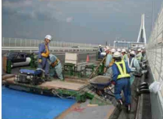
Photo 7 Provision of countermeasure for fatigue in steel deck by means of SFRC paving (blue section: epoxy resin)
