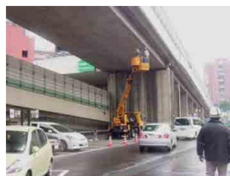
Photo 3 Close-range inspection (inspection by cherry picker; daytime inspection is available at sites where traffic flow is not adversely affected)
