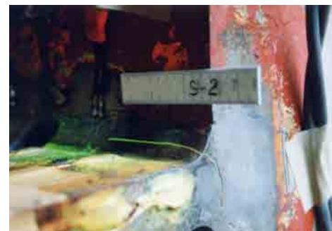
Photo 5 Occurrence of fatigue cracking (observed in weld line where beam and column cross)
