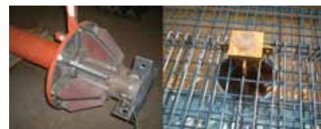
Photo 2 Example of steel capital (site welding)
