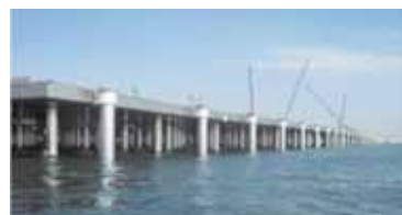
Steel pier section for New D-Runway at Tokyo International Airport
