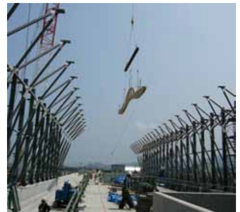
Photo 4 Hoisting of laminated member
