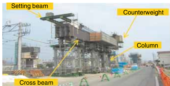
(a) Assembly of cross beam
