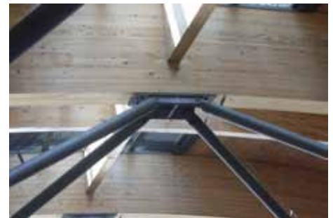
Photo 4 Laminated wood-lattice joint
