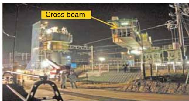
(b) Rotation of cross beam
