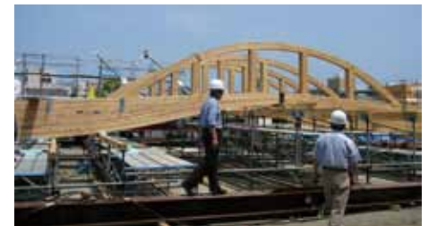
Photo 3 Ground assembly of laminated member girder
