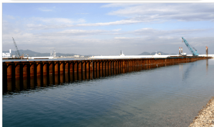
Tokushima prefecture Awazu Port sea surface disposal site (Steel pipe sheet pile)
