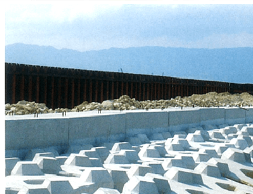
Kobe offshore disposal site (Steel sheet pile)
