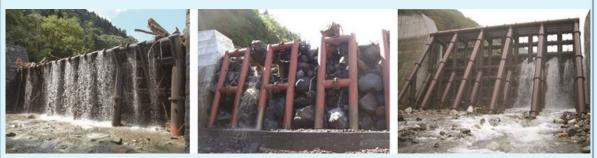
• Slit-type structure is designed considering the ecosystem, which does not disrupt river flow
