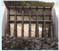
Water and harmless sediments flow down under normal conditions
