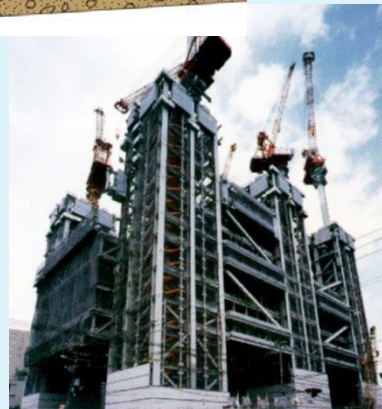
Damping structure by buckling-restraint brace
