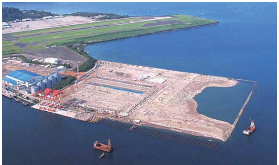
Photo 1 New Container Terminal at Cubi Point
