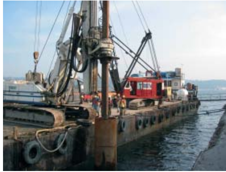
Photo 4 Pre-drilling at Marine Terminal
