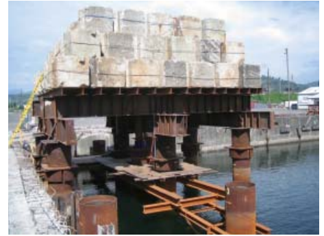
Photo 5 Static load test (Kentledge)
