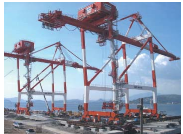
Photo 6 Quay gantry crane being unloaded
