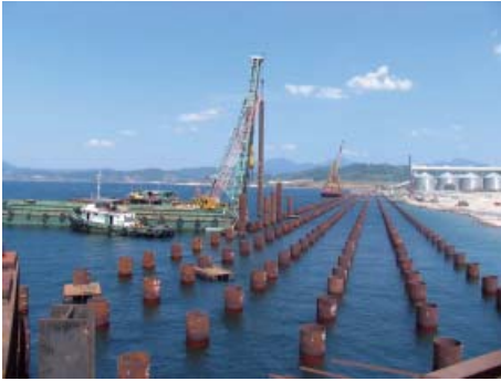
Photo 3 Pile driving at New Container Terminal
