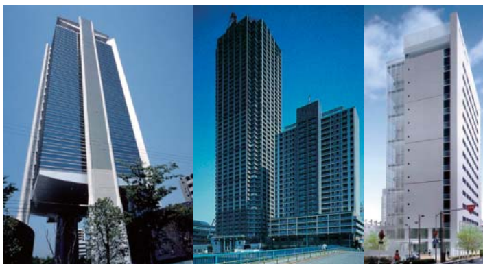
Photo 1 Examples of medium- and high-rise buildings constructed using CFT structures
