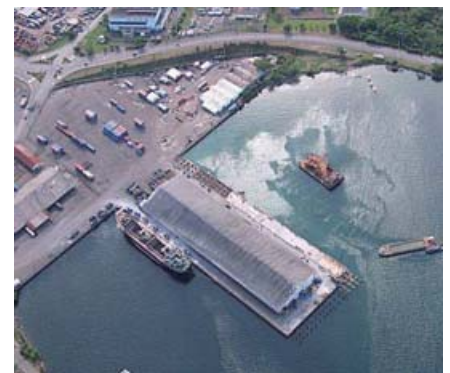
Photo 2 Marine Terminal (NSD District) — Marginal pier to the existing wharf
